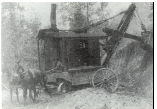
Early road construction
